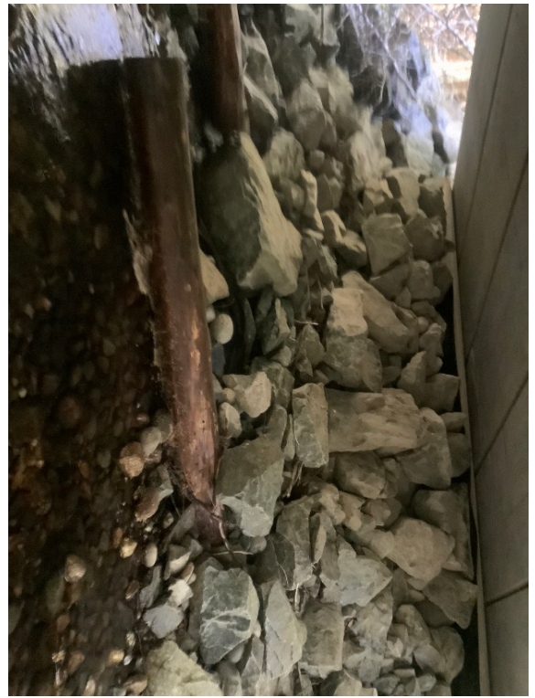
Right Bank Abutment when facing downstream
